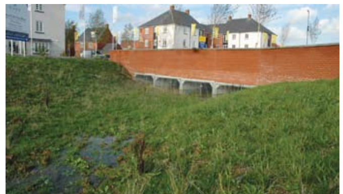
One of the three novel newt underpasses at Marnel Park
