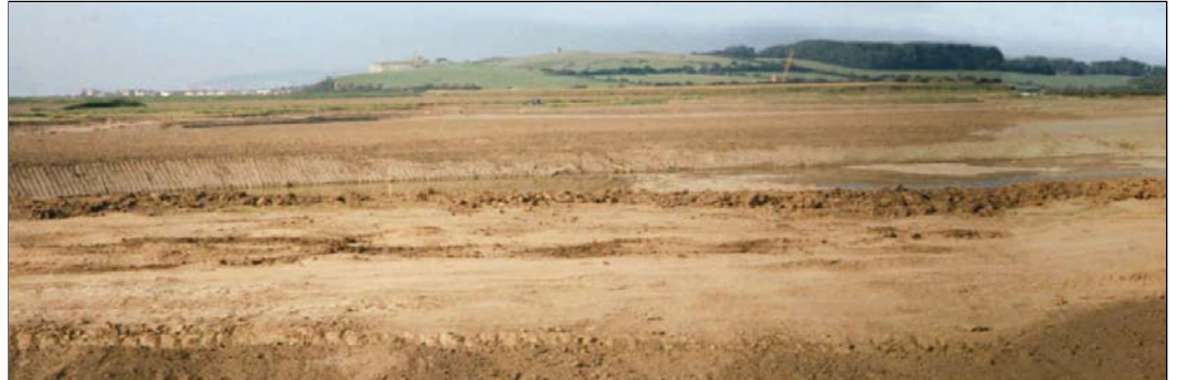
Wildlife lagoons during construction
