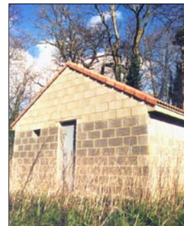
Purpose built bat roost
